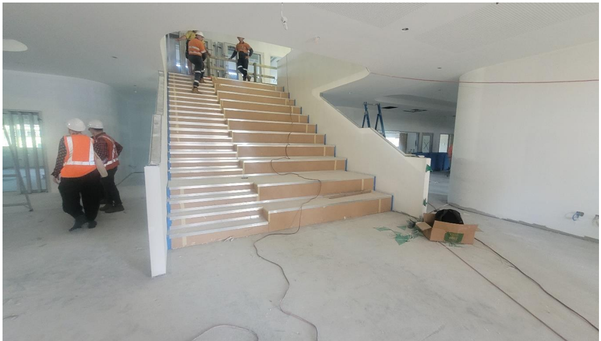
Photo 12: Internal Staircase Construction (2)
