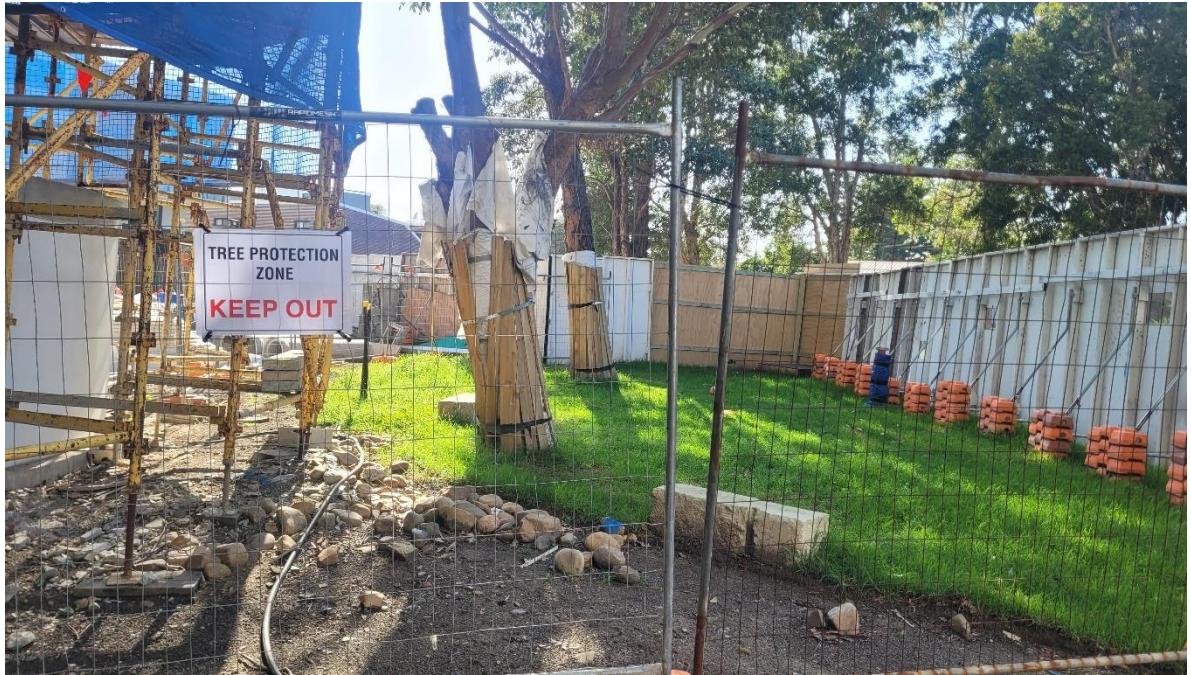
Photo 9: Tree Protection Zone (1)
