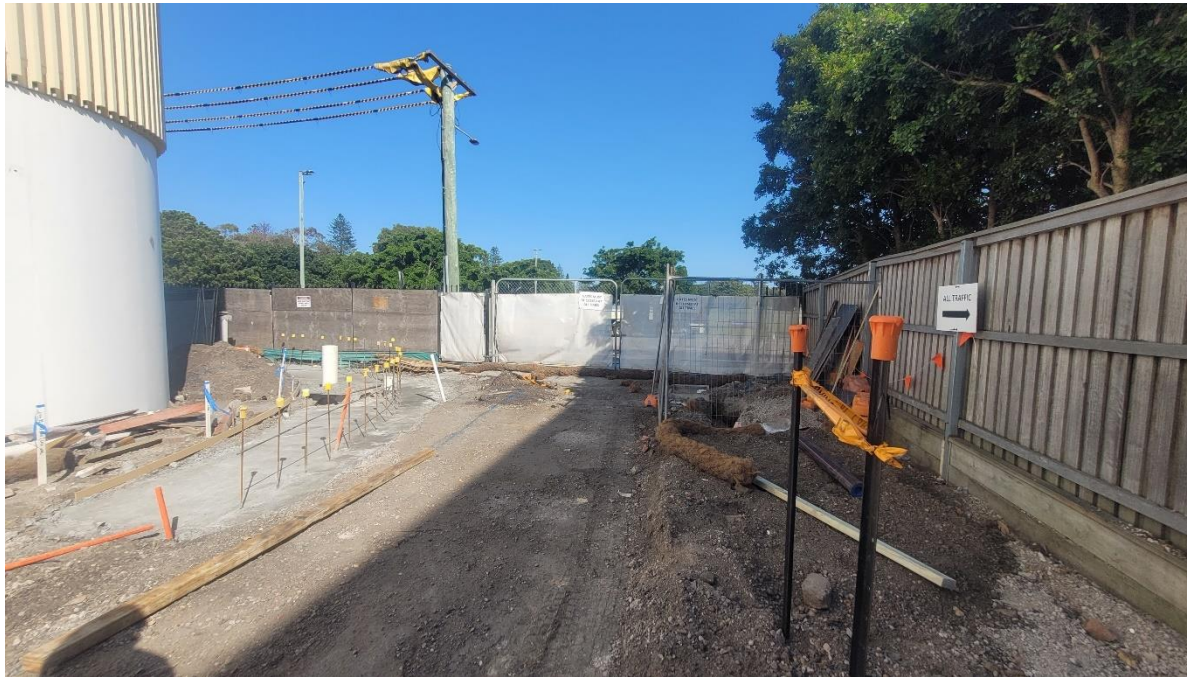
Photo 3: Union Street Site Entrance/Exit looking from within Site
