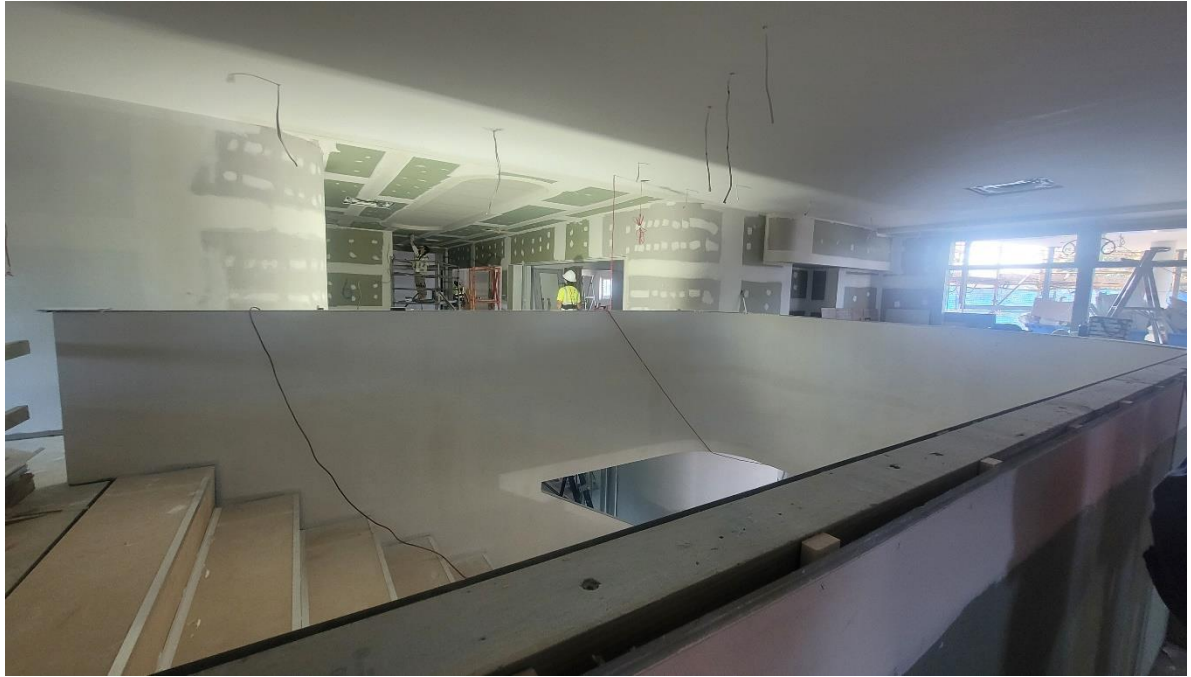
Photo 13: Internal Staircase Construction (1)
