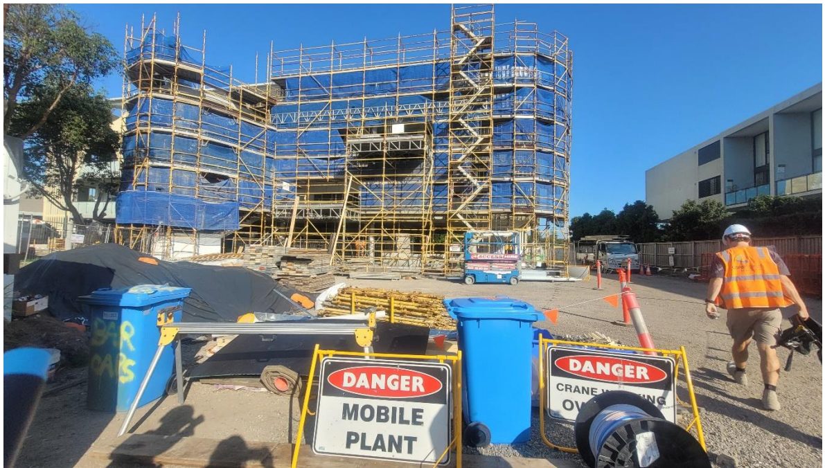
Photo 6: Stage 1 Union Street Building looking towards Union Street
