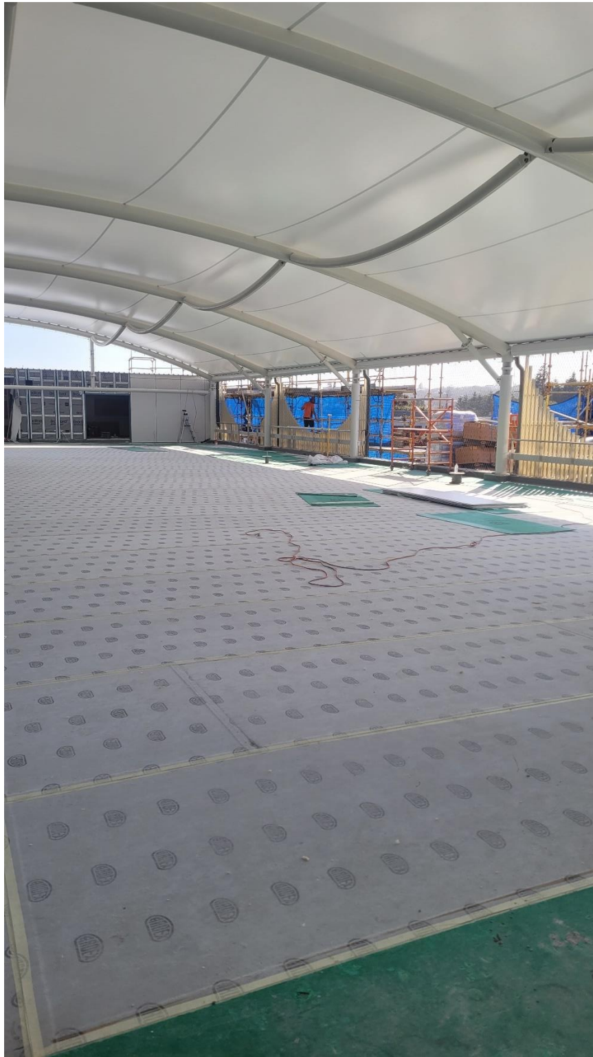
Photo 14: Top floor Construction
