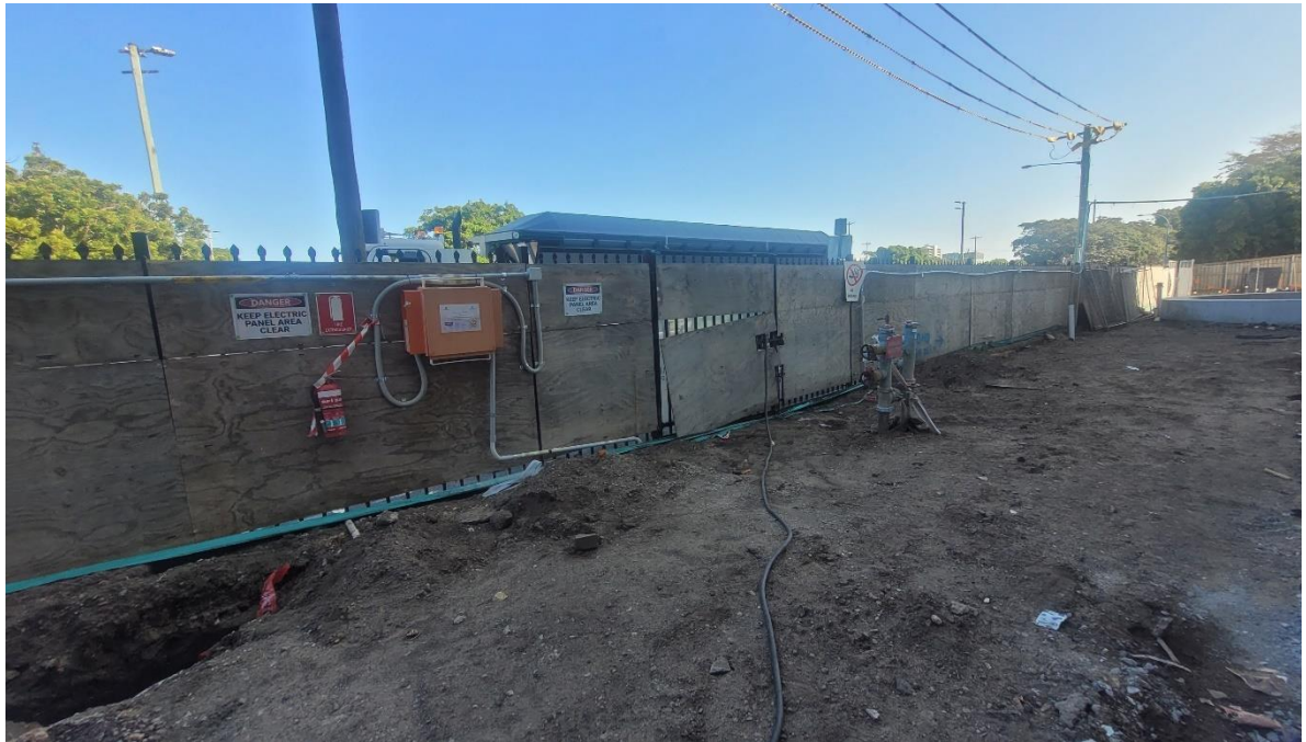
Photo 7: Site fencing looking towards Union Street
