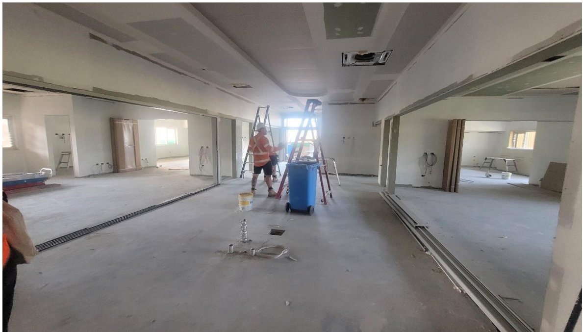
Photo 12: First Floor Construction
