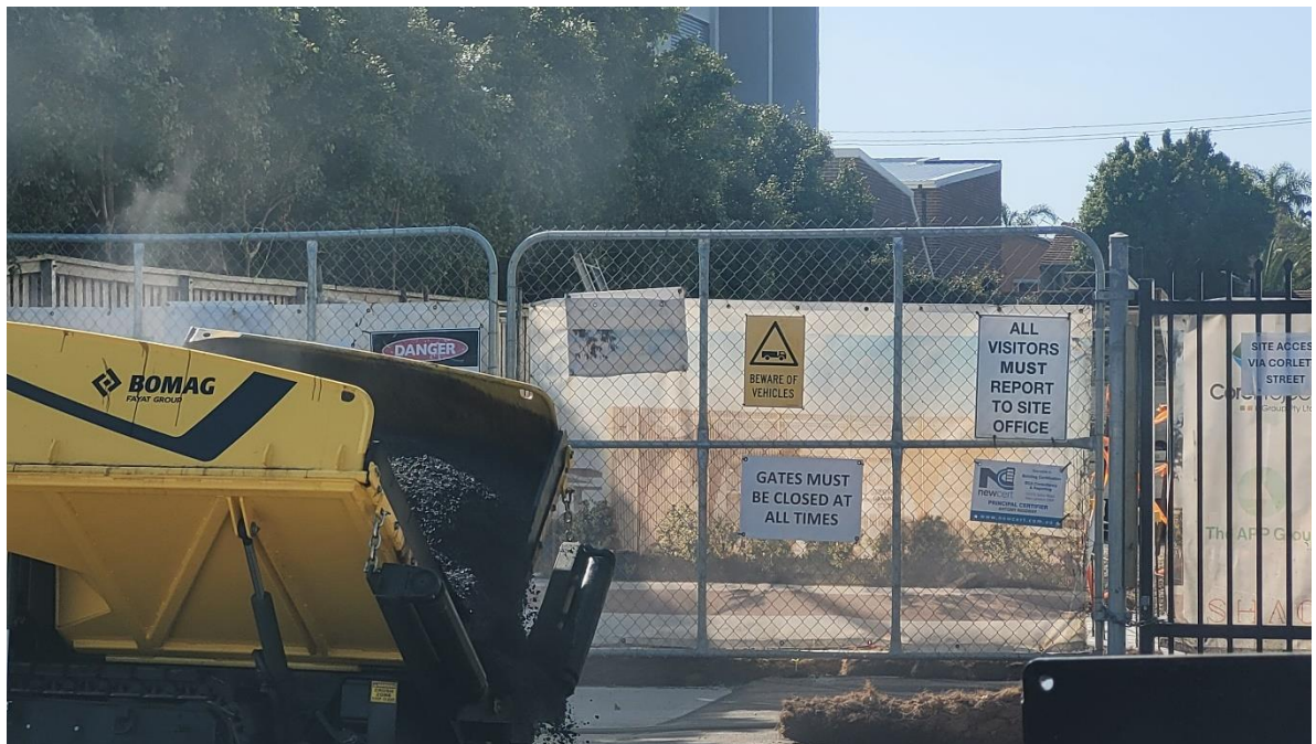
Photo 2: Union Street Site Entrance/Exit
