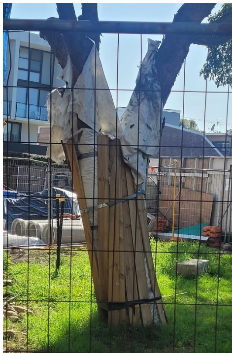
Photo 10: Tree Protection Zone (2) showing tree hoarding
