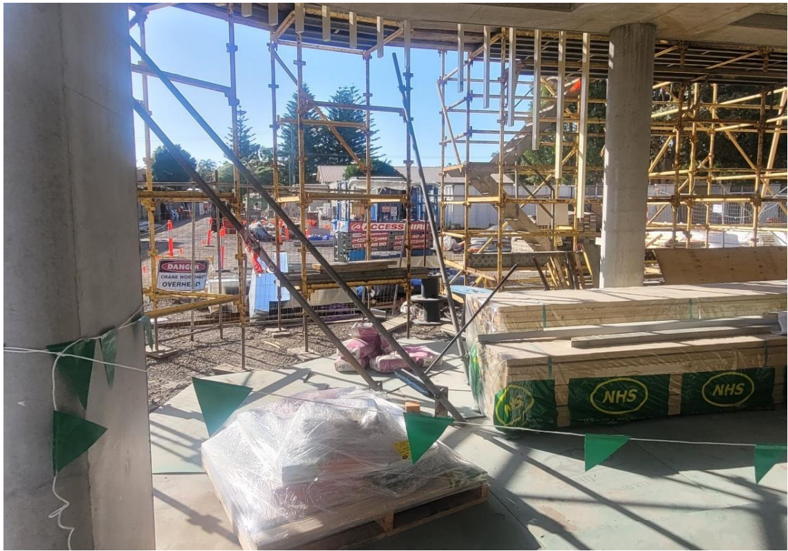
Photo 11: Ground Floor Construction
