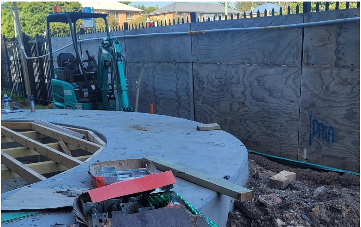
Photo 8: Site fencing looking towards Union Street
