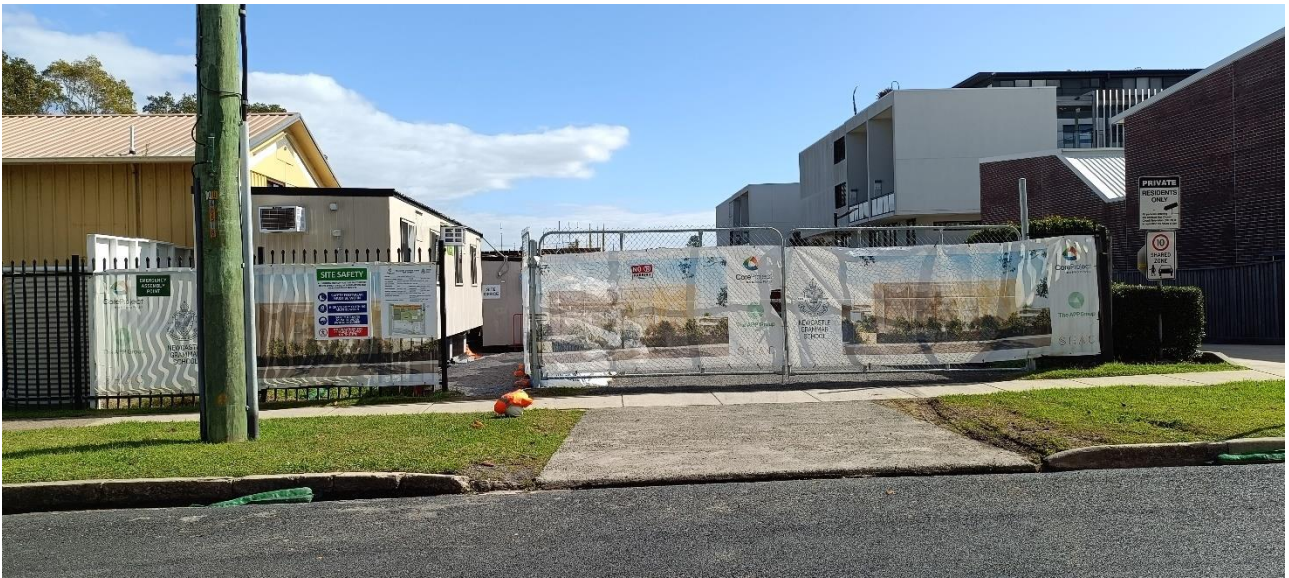
Photograph C.3 Corlette Street Gate
