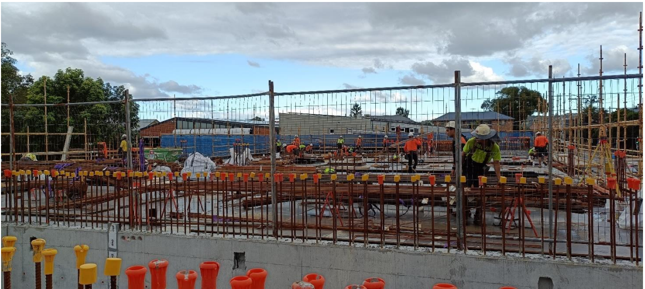
Photograph C.7 Formwork ready for concrete pour
