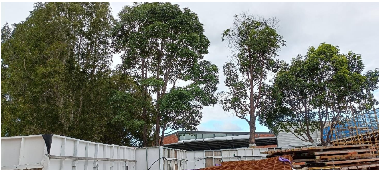
Photograph C.8 Hoarding and tree protection in place
