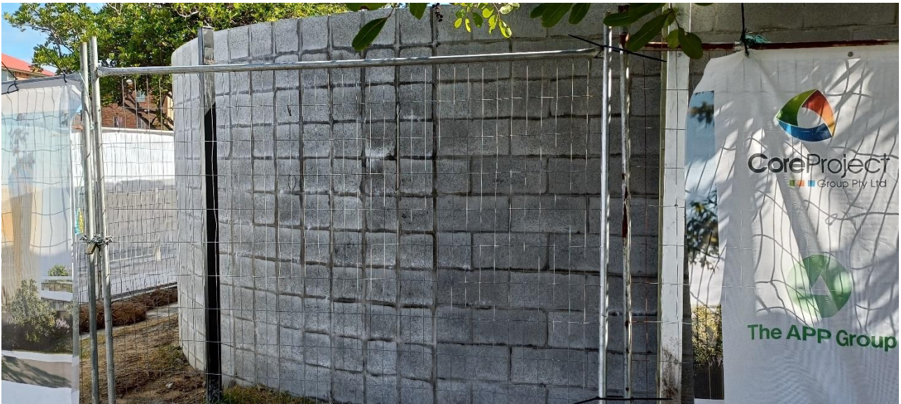
Photograph C.12 Block work fence corner of Corlette and Parkway Avenue
