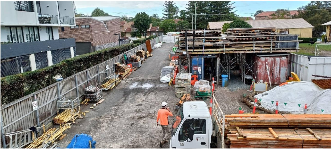
Photograph C.10 View looking east from Union Street Gate to Corlette Street Gate
