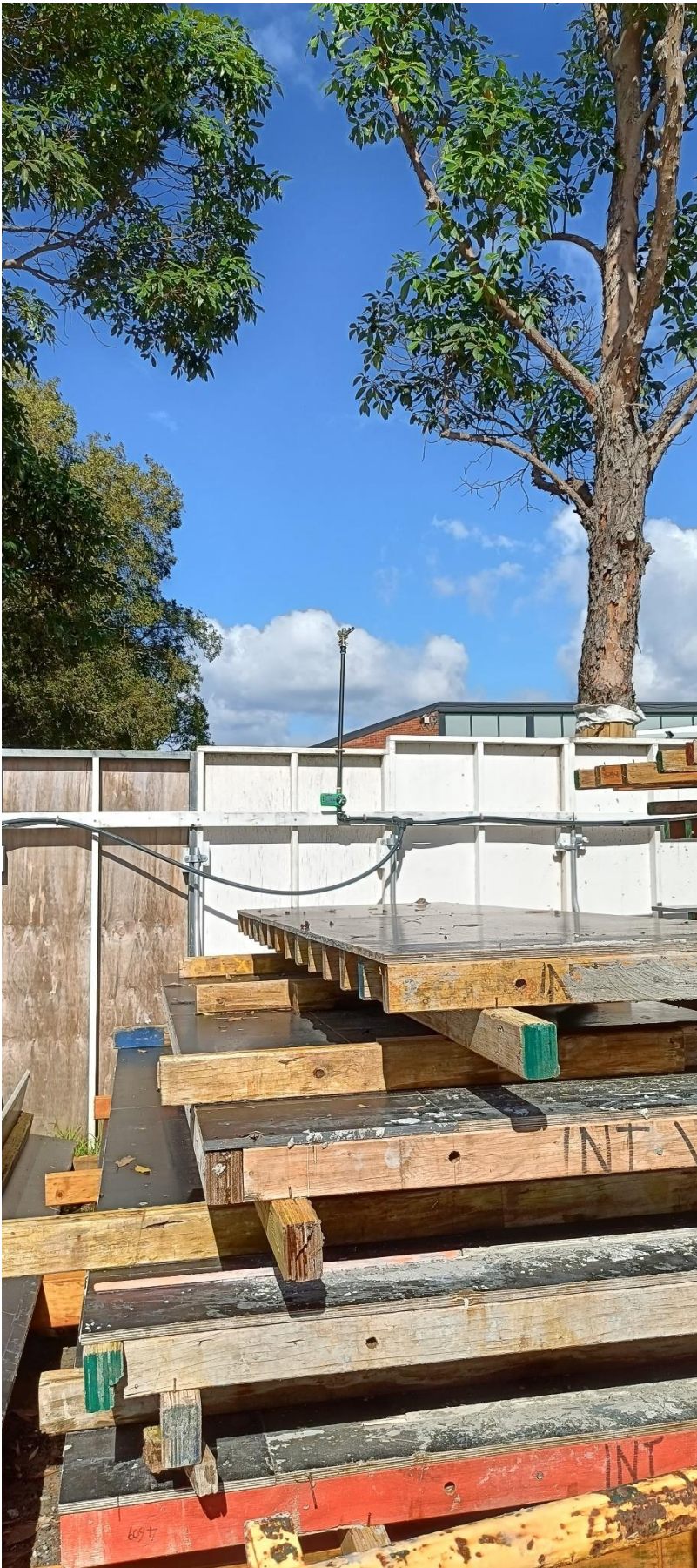
Photograph C.11 Dust suppression sprinklers in place along fence line.
