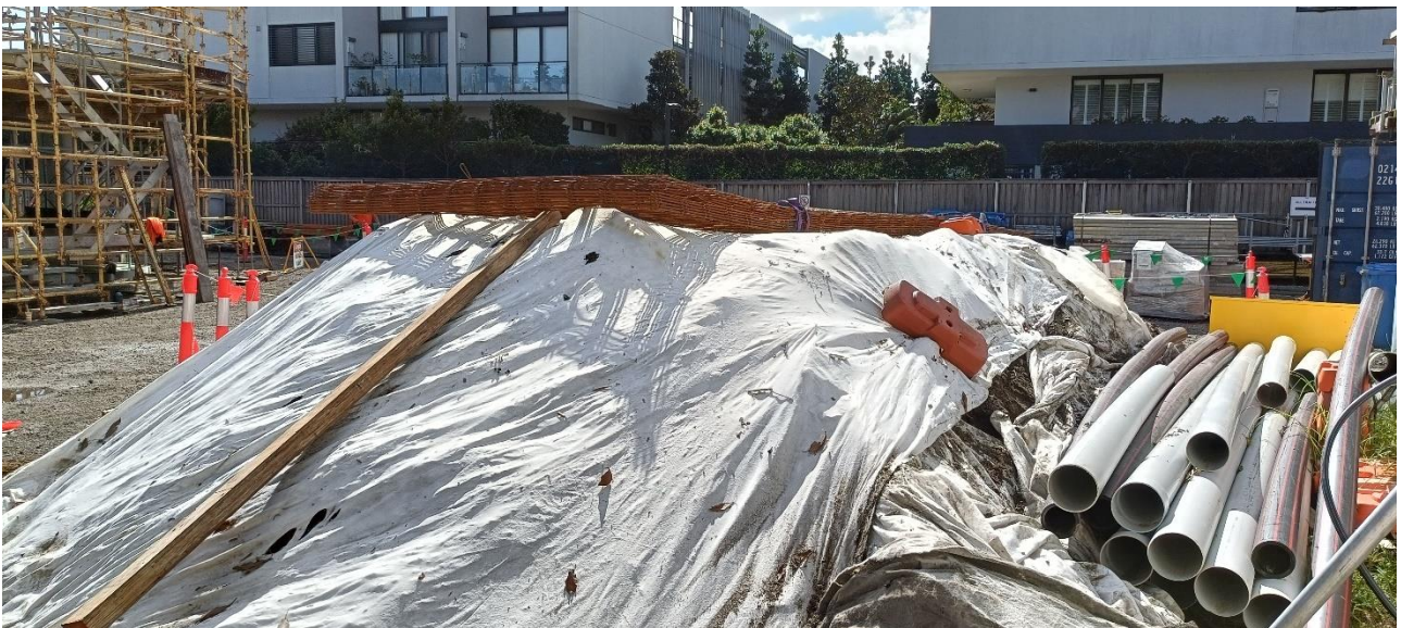
Photograph C.4 Excavated spoil material awaiting contamination testing and classification for disposal
