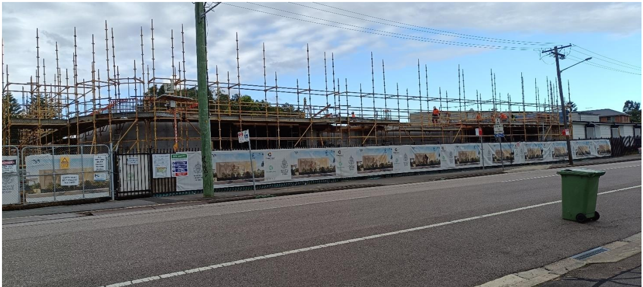
Photograph C.2 Fence wrapping – Union Street
