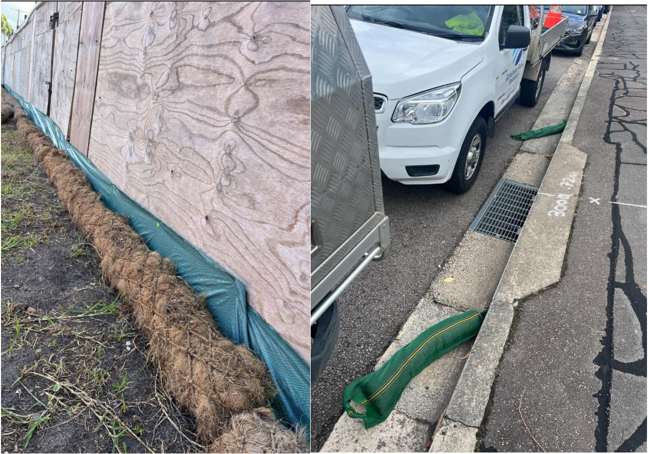
Photograph C.12 Erosion and sediment control installation (pre-construction CoreProject team)
