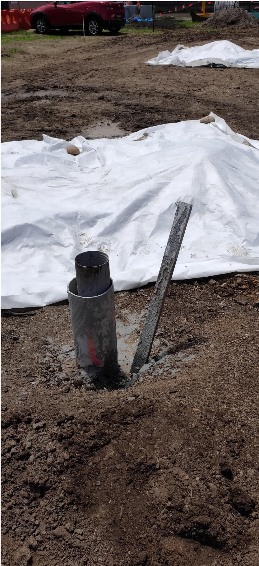
Photograph C.10 Mine Void grouting works borehole
