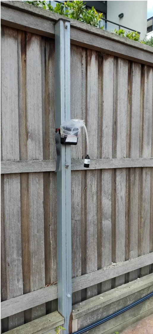
Photograph C.8 Air monitoring during archaeological salvage and grouting works
